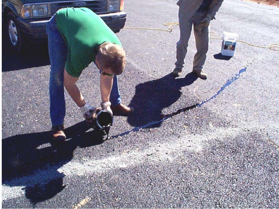
Photo 21. Pouring polymer-modified binder into probe trench
