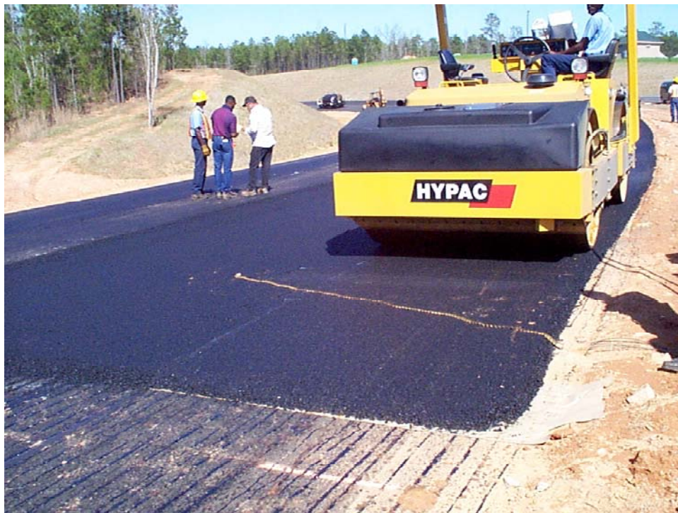
Photo 16. Compacting ropes into asphalt concrete to form temperature probe trenches
