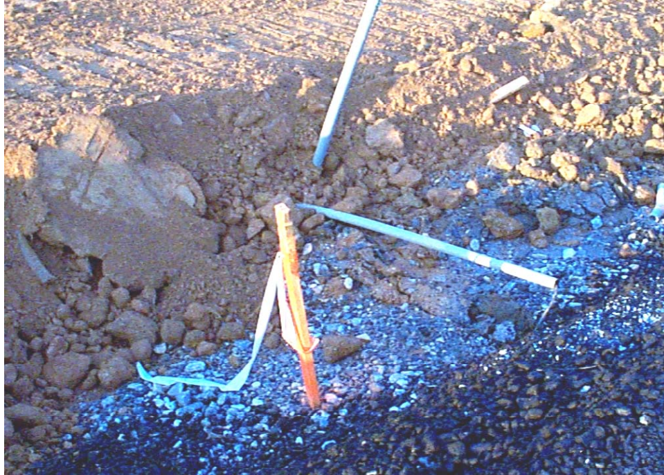
Photo 15. Moisture probe cable threaded through PVC pipe, extending through pavement shoulder
