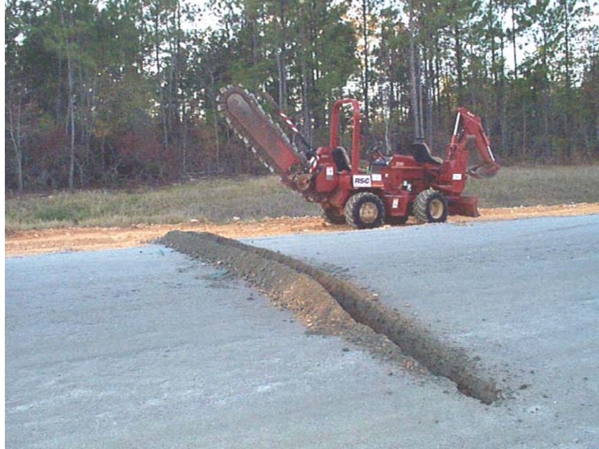
Photo 10. Trench for installing a CS615 moisture probe
