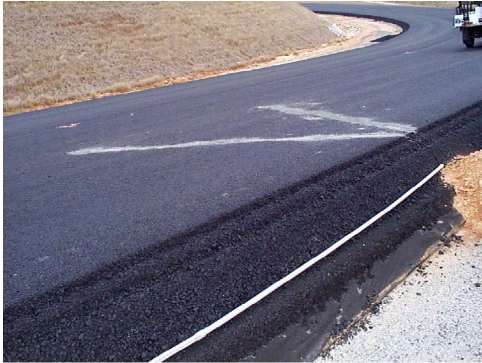
Photo 23. Completed temperature probe installation on top of the upper binder course
