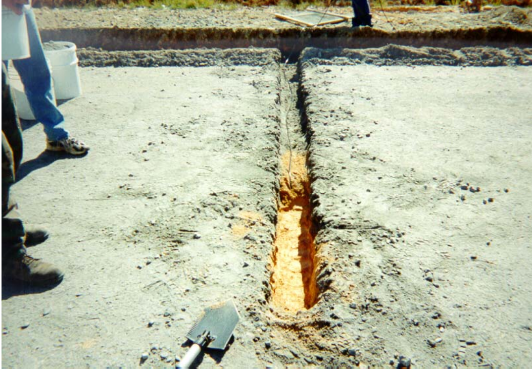
Photo 13. CS615 probe installation after compacting select fill
