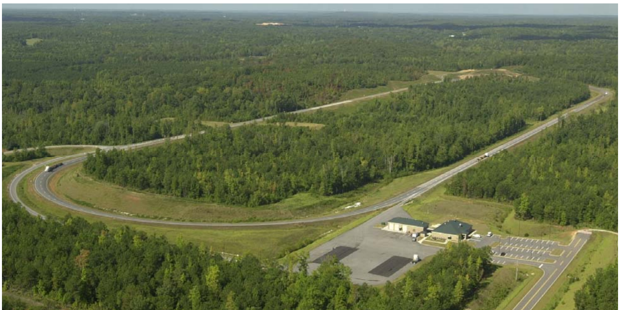
FIGURE 1 Aerial Photograph of NCAT Pavement Test Track
