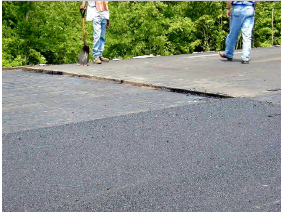
Figure 16. Transverse Joint and Tack Coat Preparation.
