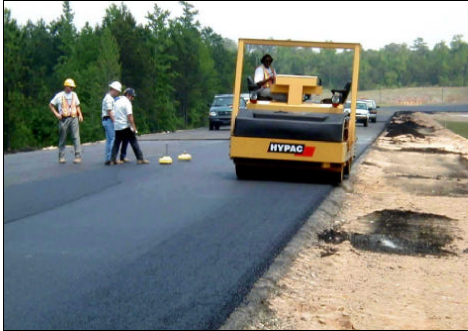
Figure 21. Hypac C778B Vibratory Double Drum Compactor and Density Monitoring.
