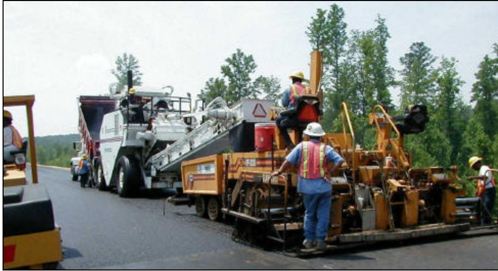
Figure 17. Loading, Material Transfer, and Laydown Operations.
