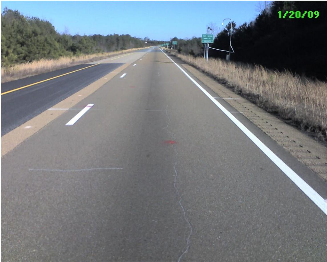
**FIGURE 7.1 Cracking Severity in Section S2 after 30 Million ESALs.**
