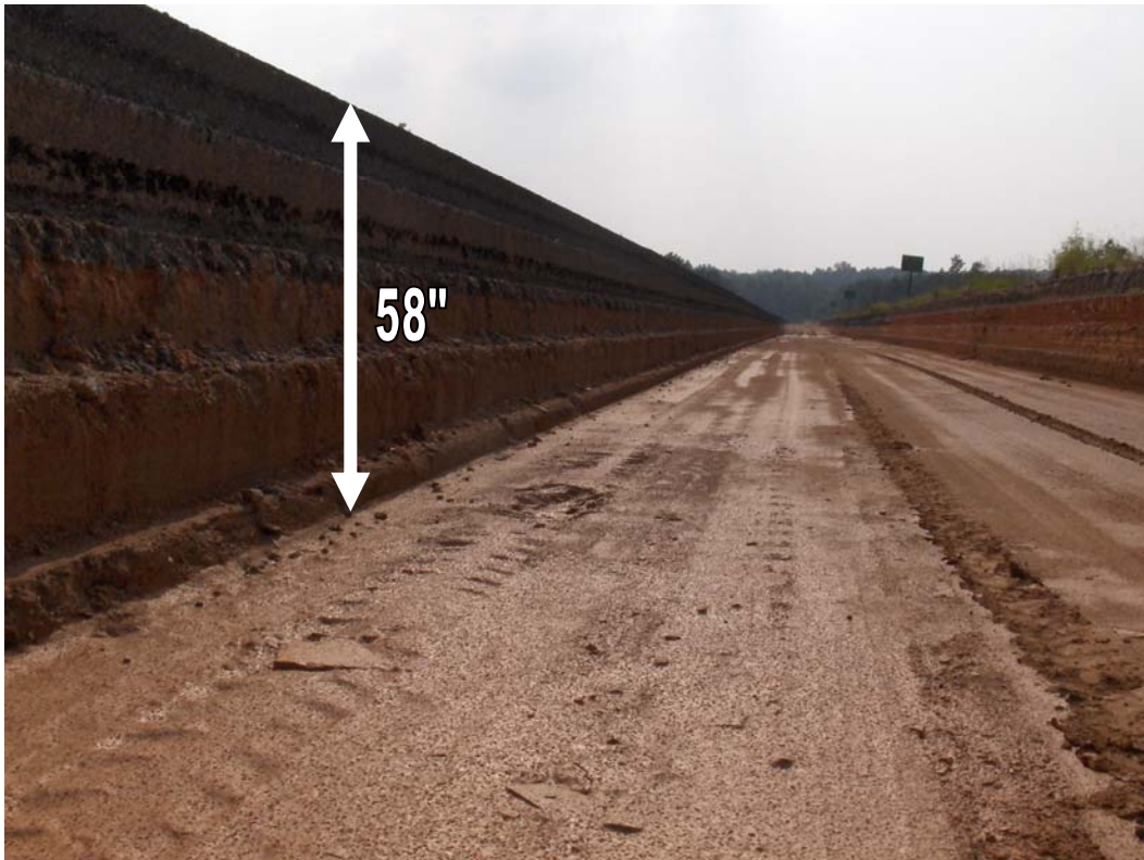
Figure 4.2 Section N8 at Conclusion of Pavement Removal (8/24/2006).
