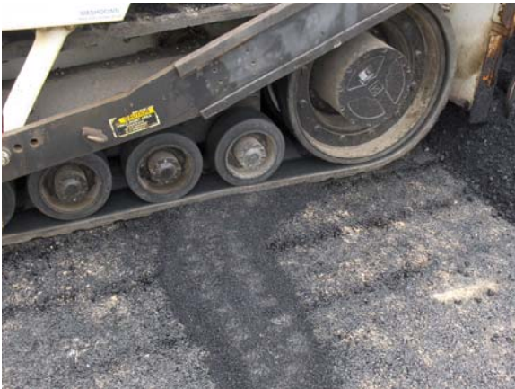
c. Paver Crossing Over Gauge Cables.
