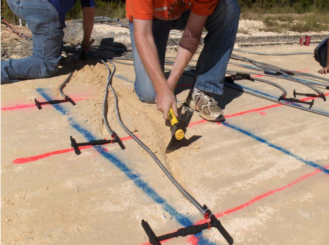
Figure 4.16 Preparing Trenches for Cables in Aggregate Base.
