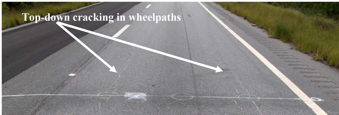
Figure 2.2 Top-Down Cracking in Section N5.
