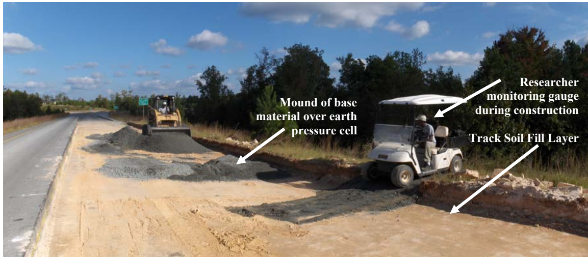
Figure 4.11 Placing Aggregate Base in Section S11.
