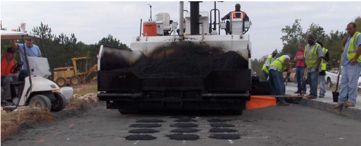
Figure 4.20 Paver Approaching Gauge Array (S11).
