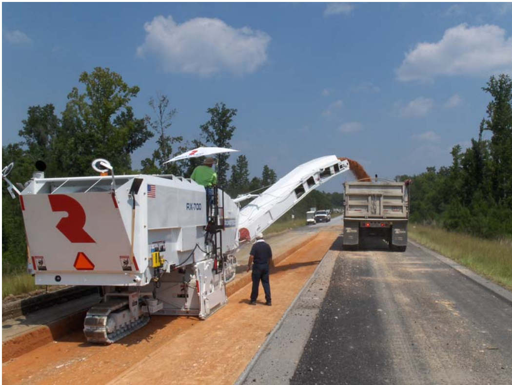
Figure 4.1 Milling Operation in Section N8 (8/18/2006).
