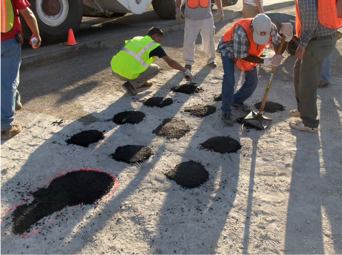
Figure 4.19 Placing Cover Mix (N10).
