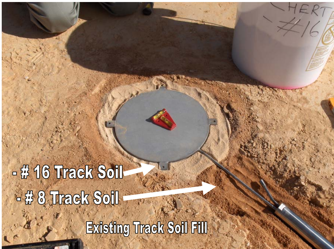
Figure 4.9 Installation of Fill Pressure Cell in Section S11.
