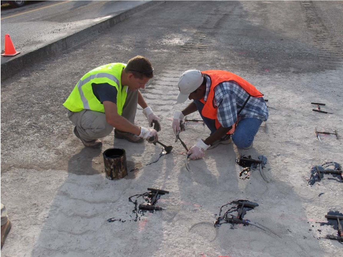
Figure 4.18 Tacking ASG's into Place (N10).
