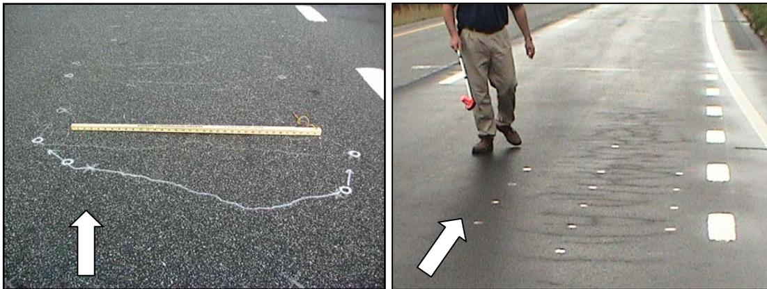
**Figure 5.18 Progressed Fatigue Cracking.**
