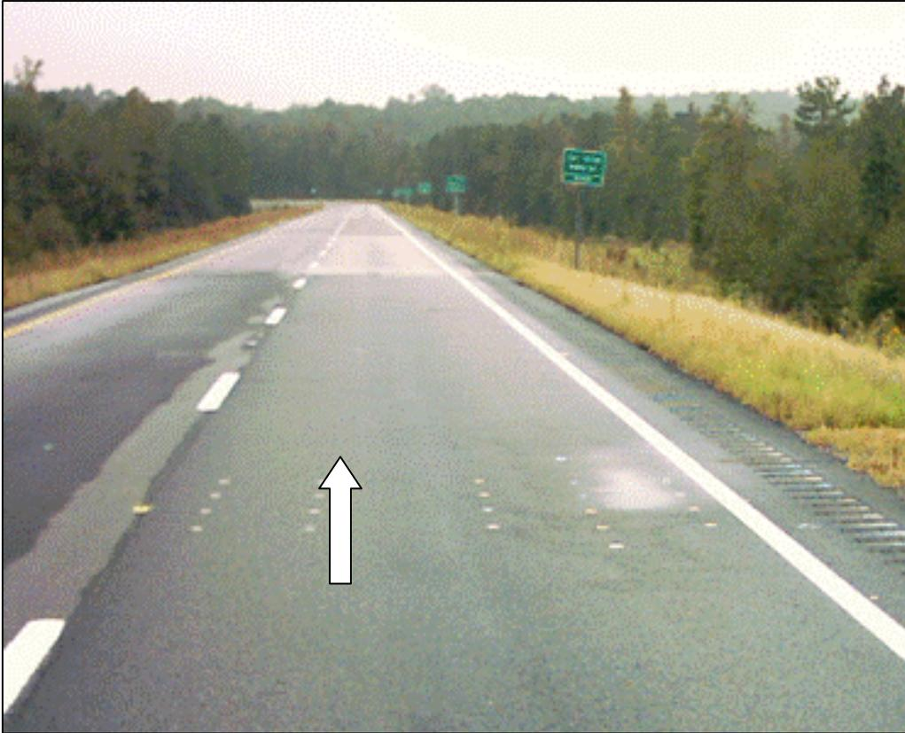
**Figure 5.19 Water Ponding Due to Rutting– Section N8.**
