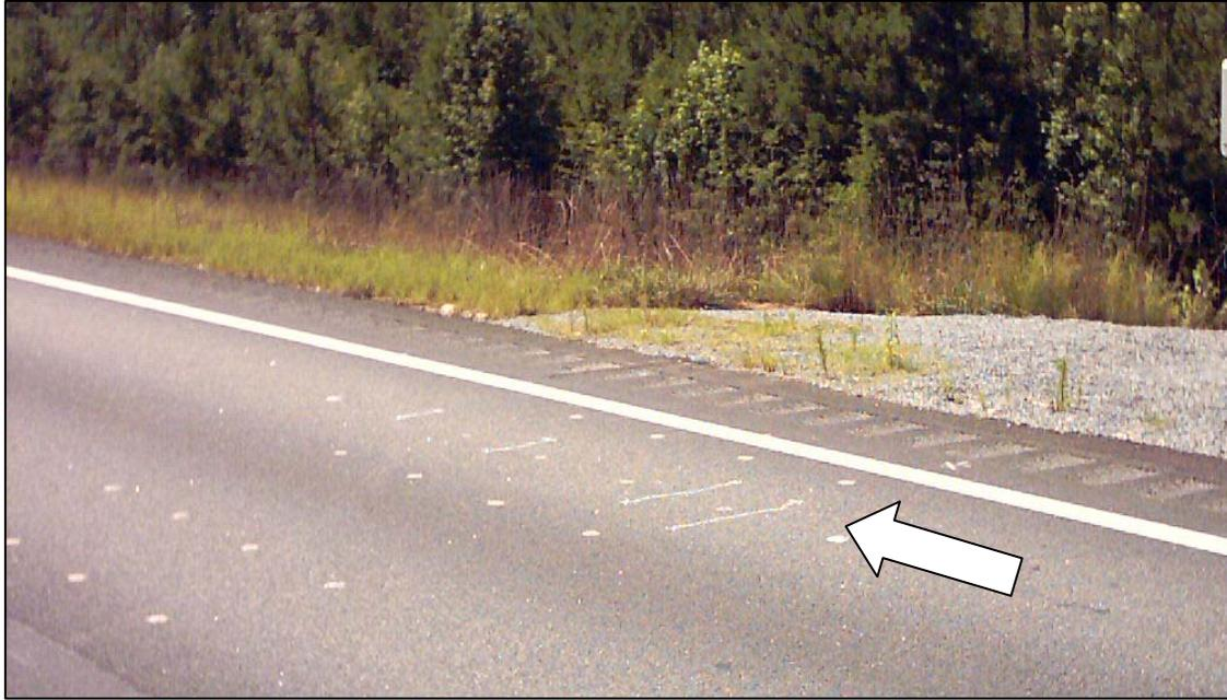
**Figure 5.17 Transverse Cracking in Wheelpath - Section N8.**
