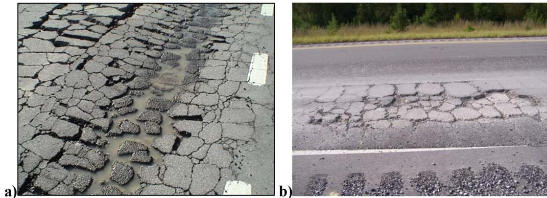
**Figure 5.20 Extensive Fatigue Cracking in Section a) N1 b) N2.**
