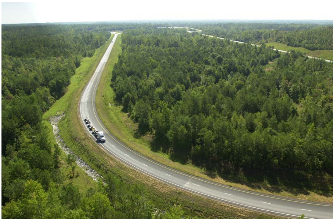
Figure 3. NCAT Test Track.
