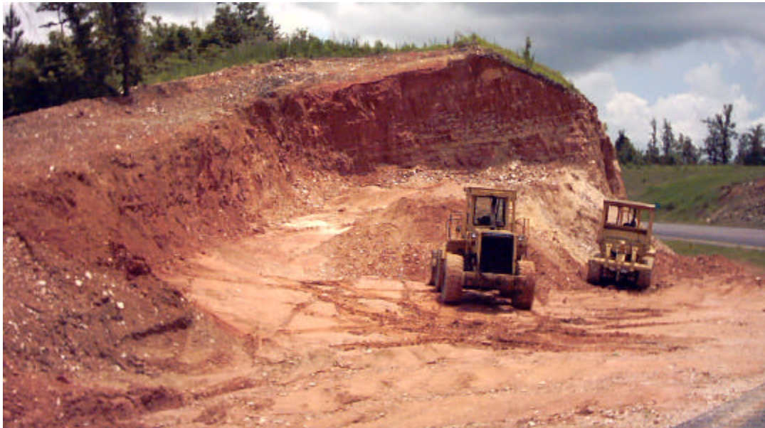
Figure 17 – Onsite Source for Structural Subgrade Material
