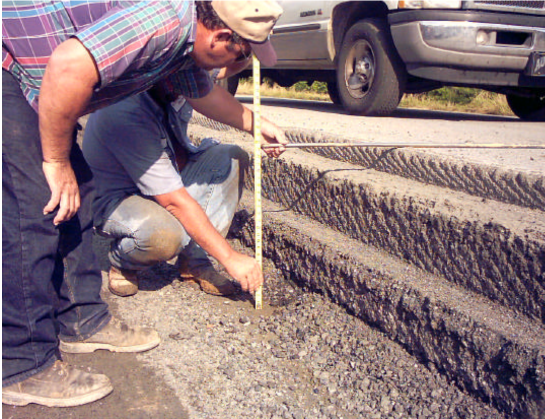
Figure 16 – Completed Deep Milling of Hot-Mix Asphalt Layers
