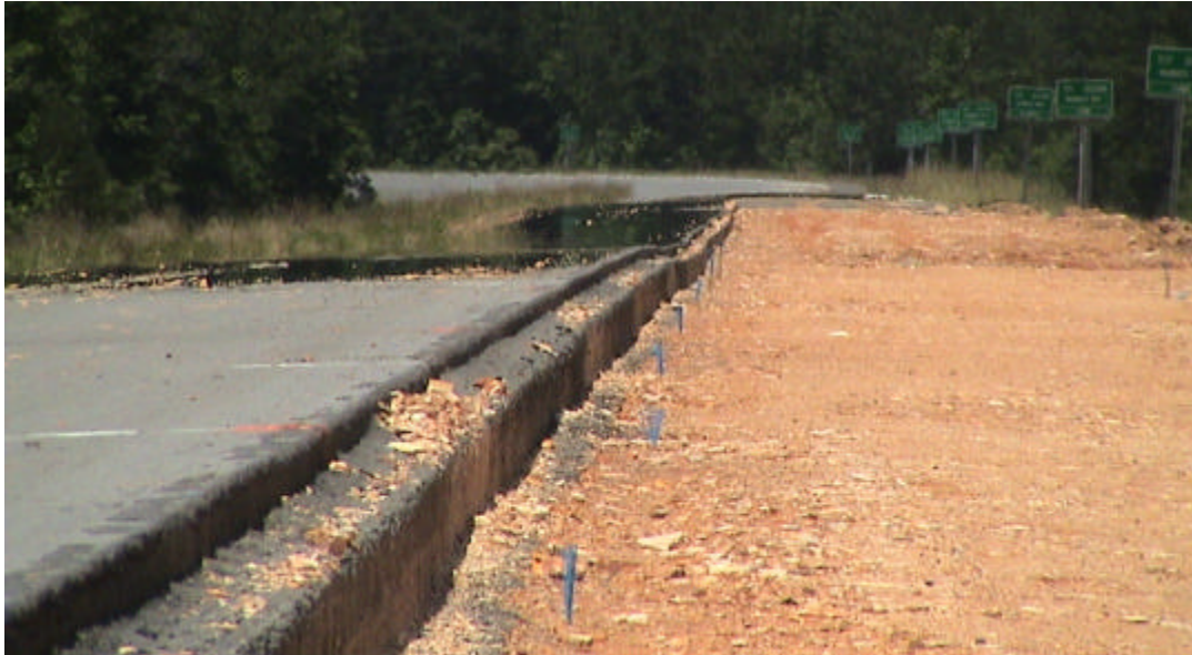
Figure 19 – Visually Discernable Settling of North Tangent
