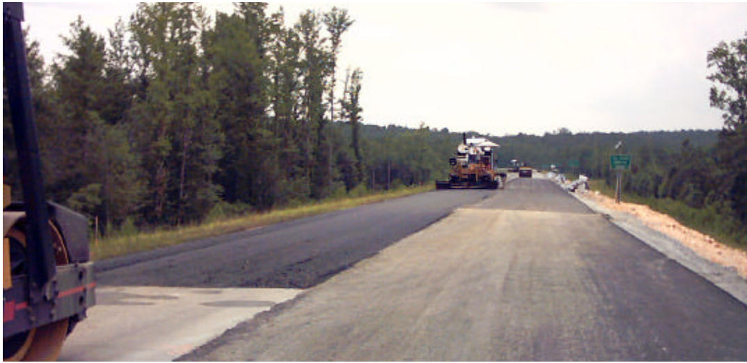
Figure 21 – Inside Lane Leveling for Settlement Mitigation
