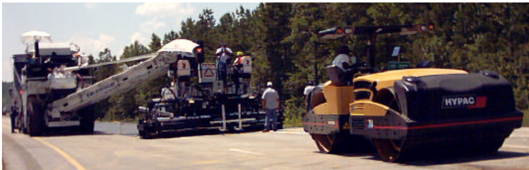
Figure 9 – Preparing to Pave a Test Section with Aggressive Rolling
