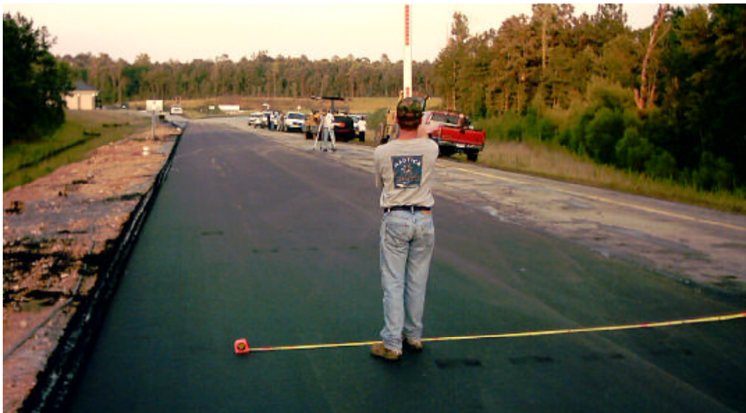
Figure 22 – Wheelpath Survey to Fine Tune Screed Placement Thickness
