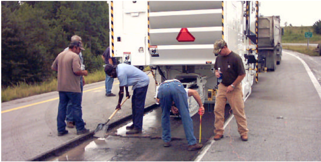
Figure 23 – Detailed Mill Thickness Verification
