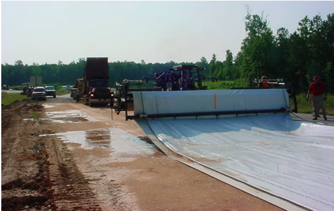
Figure 18 – Tarping System Utilized During Subgrade Construction
