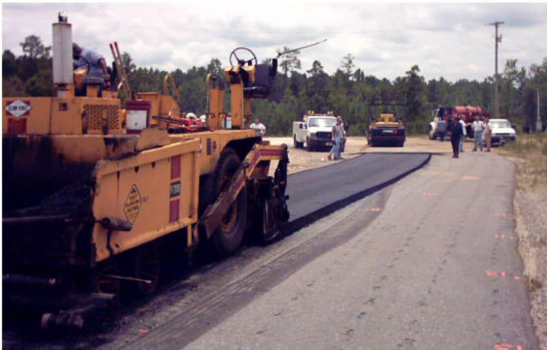
Figure 7 – Paving Trial Mix Before Placement on Track
