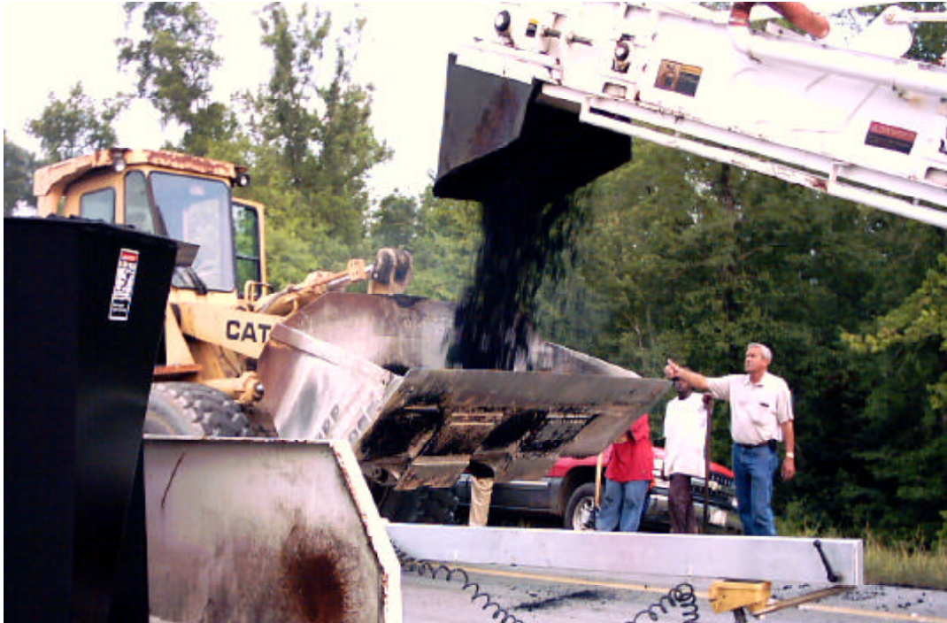
Figure 12 – Sampling Representative Research Mix from Roadway
