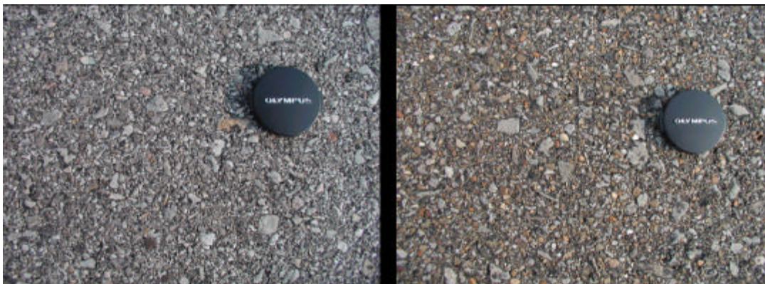
Figure 32 – Oklahoma’s Traffic Only Mixes (Hveem Left, Superpave Right)
