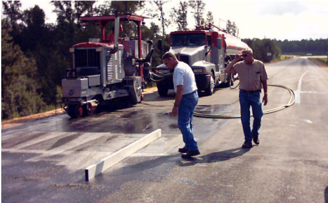
Figure 13 – Diamond Grinding Select Sections for Smoother Joints
