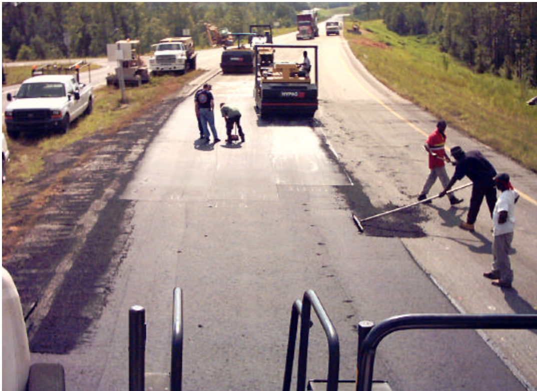
Figure 25 – Construction of Florida Test Section
