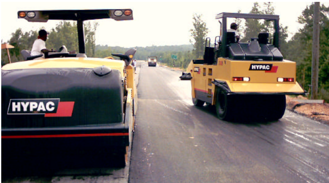
Figure 11 – Pneumatic Rubber-Tired Rolling in Intermediate Temperatures
