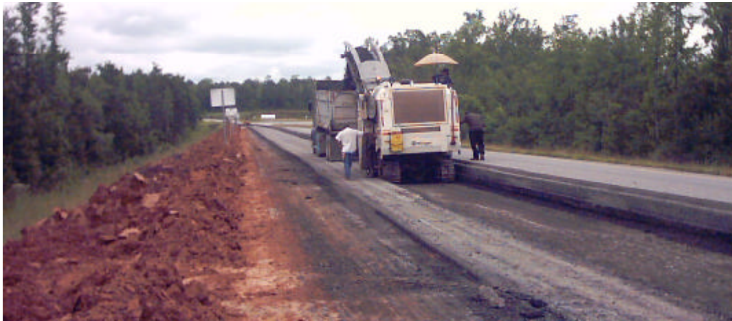
Figure 15 – Deep Milling to Remove Existing Pavement Structure
