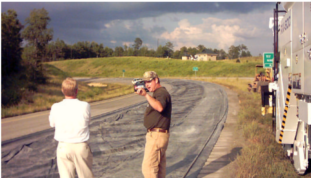
Figure 24 – Weather Protection for Milled Rutting Sections
