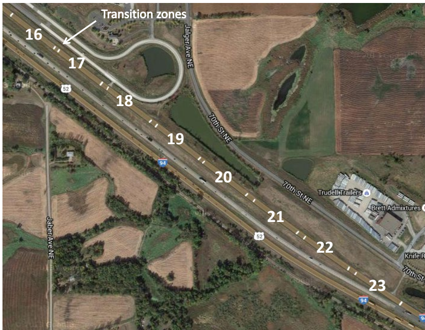
Sections 16-23 (8 test sections)
