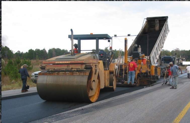
Mix placed at 3:15 PM
