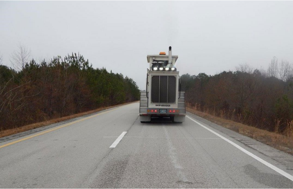
Shotblasting S7A & S7B
