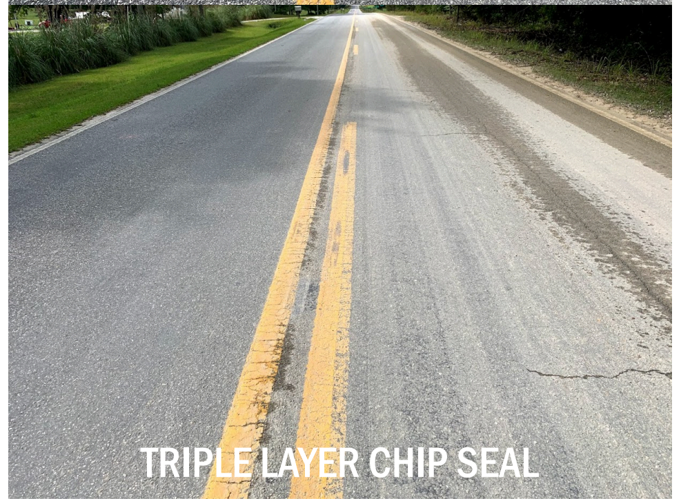
FIBERMAT CHIP SEAL
