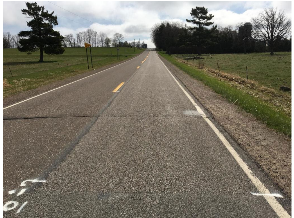
FIBERMAT CHIP SEAL
