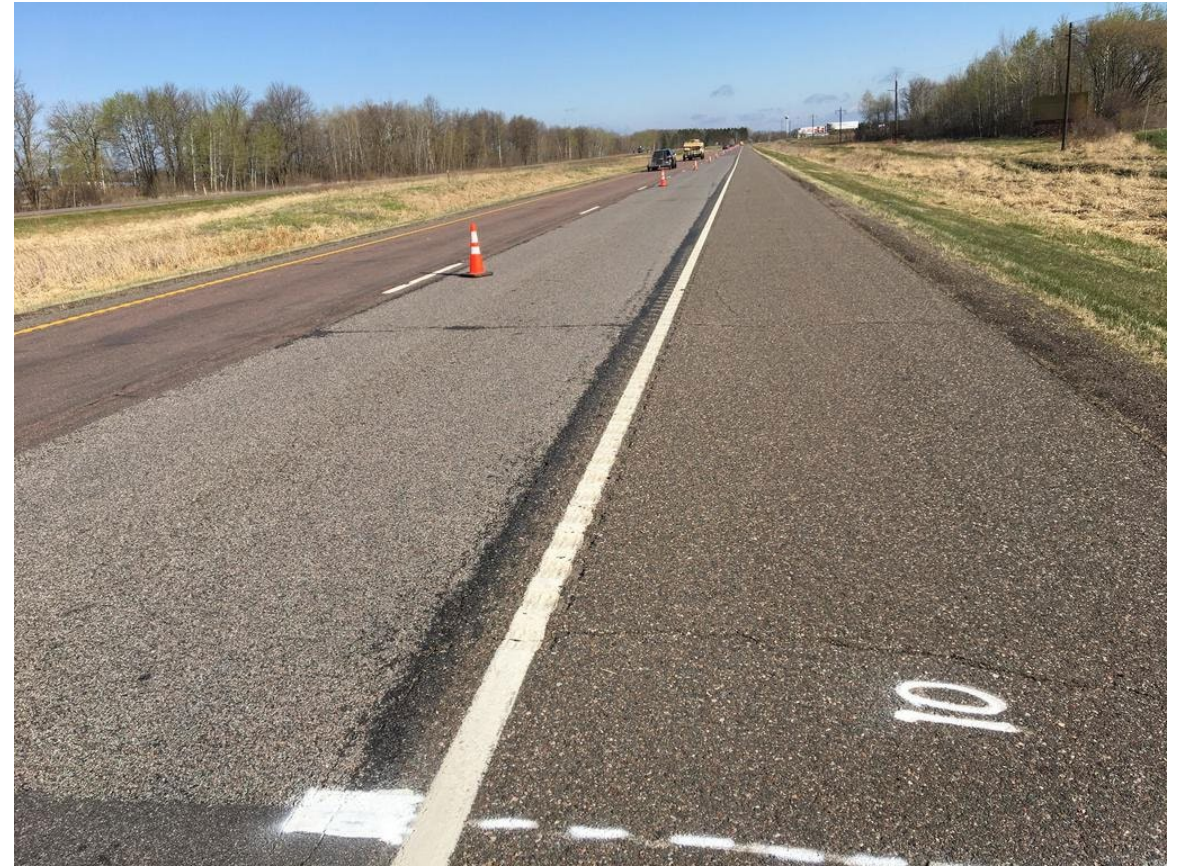
FIBERMAT CHIP SEAL
