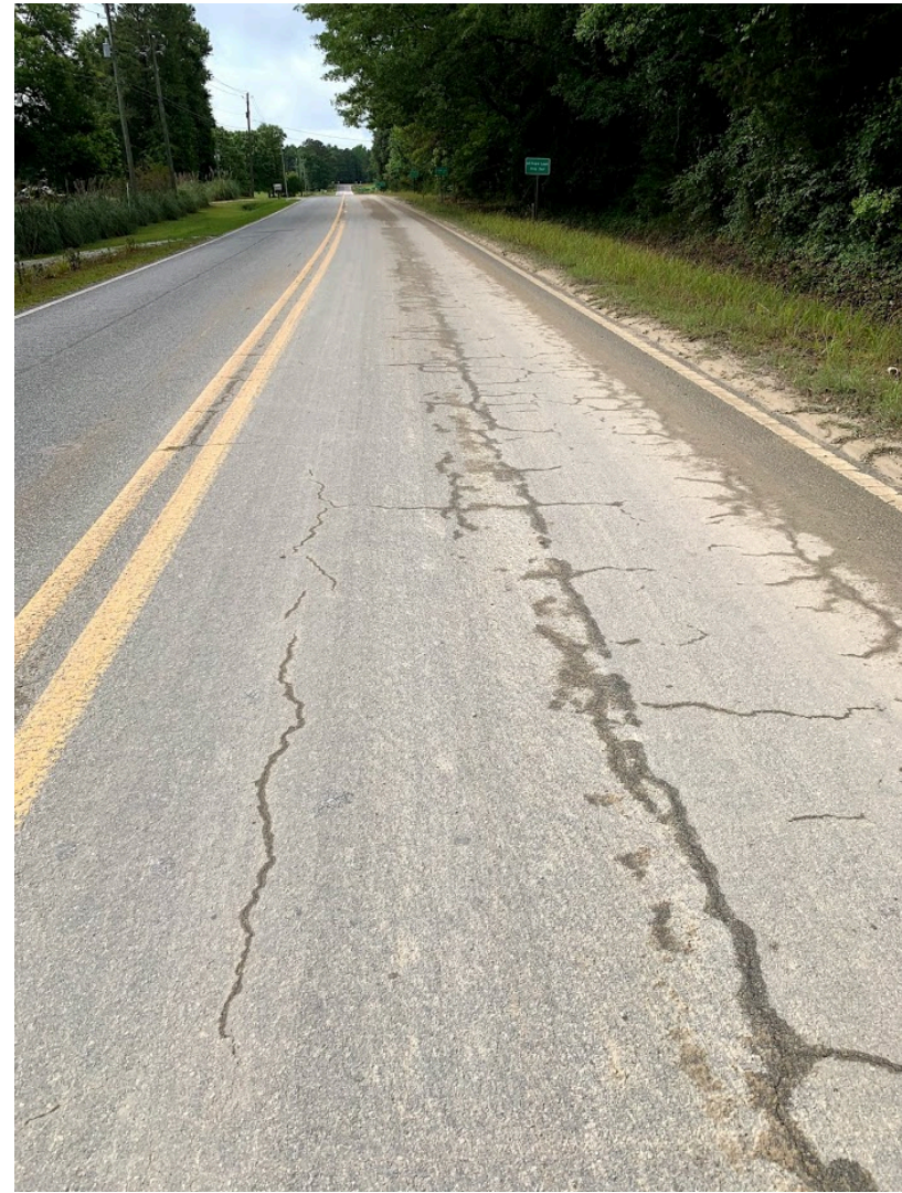
SINGLE LAYER CHIP SEAL + CRACK SEAL
