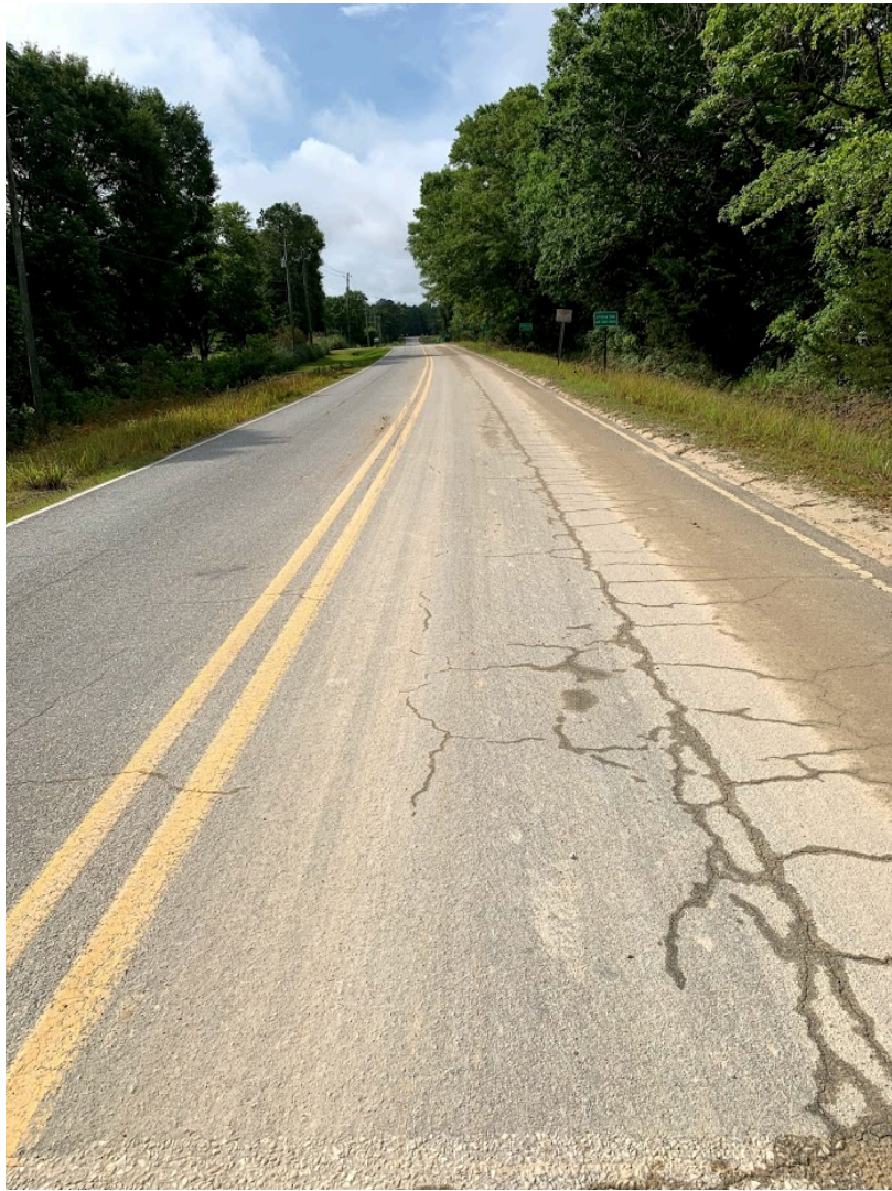
SINGLE LAYER CHIP SEAL
