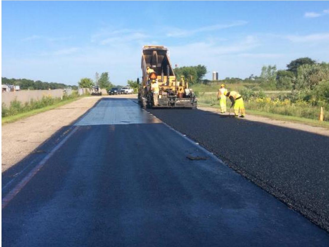
August 2016 – Hardrives Contractor
