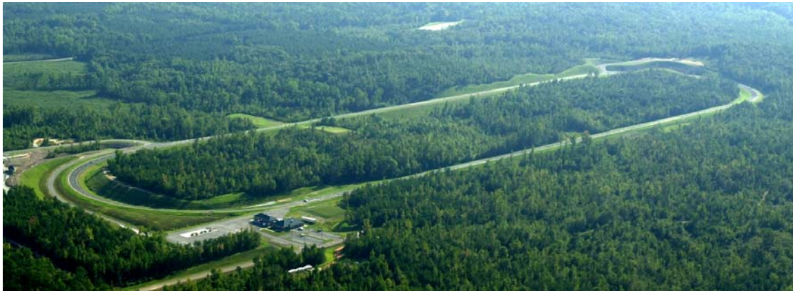
Figure 6 – Pavement Test Track at Auburn University
